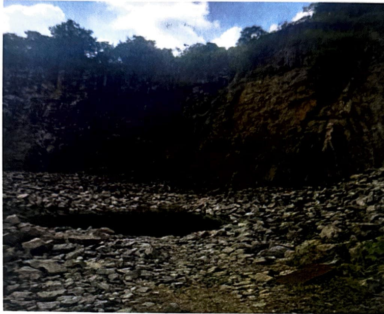
Fig..3 View of the sub-vertical face of the old quarry pit awaiting closure. Though there are damp patches on the lower part of the cliff, distinct seepage of water was not seen. However, through a depression on the top, storm water from the upper road section was found to enter into the pit creating a pool of water in the central part.
